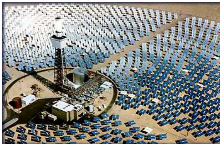
A field of PV's gathering sunlight to produce power
